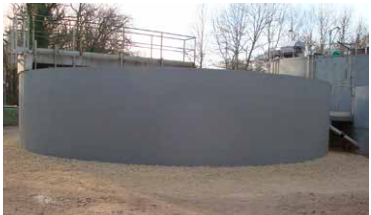
Completed work, not a day's interruption.
